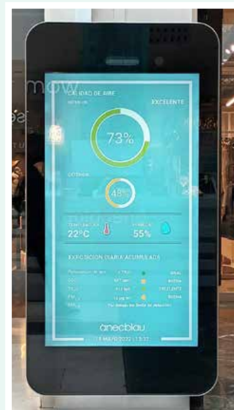
Air quality control at the Ànec Blau shopping centre (Barcelona)
