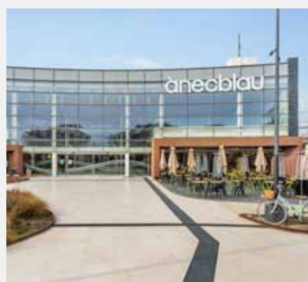
Ànec Blau: completing the façade and adding a new outdoor food court area.
