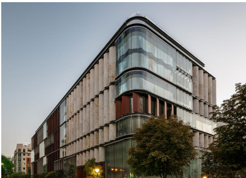
Façade from Calle Juan Bravo
