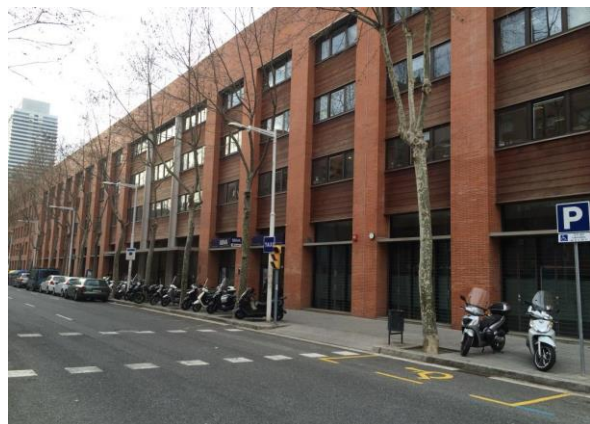
Aerial and front views of the building acquired
