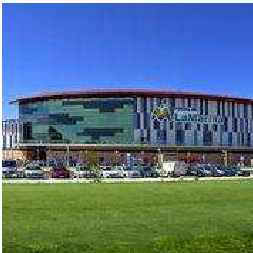
Outside Facade of the Building
