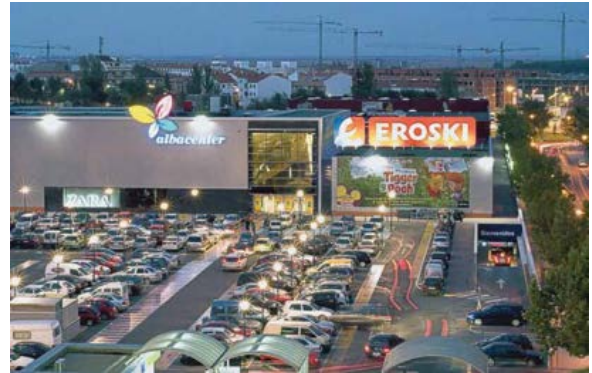
Parking Exterior del Centro Comercial
