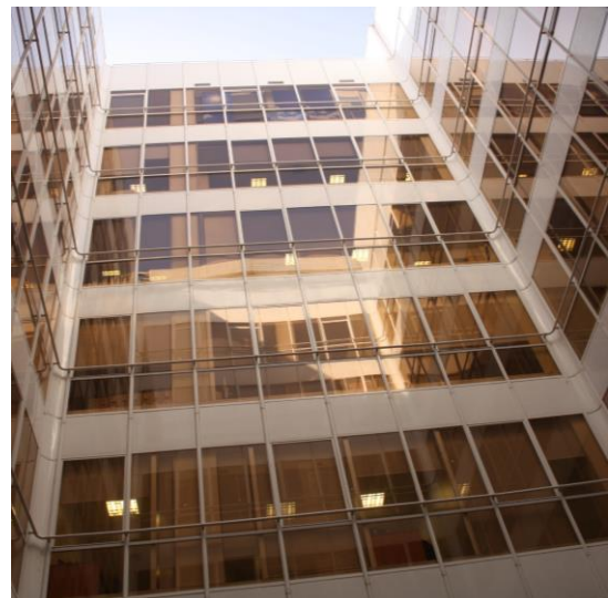
Inside View of the Building
